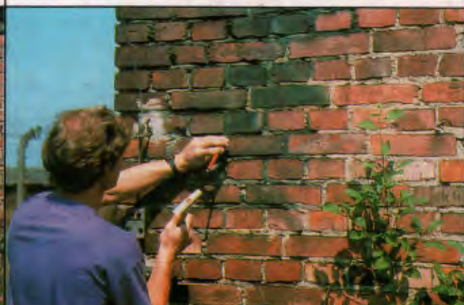
Illustration 11: Even the outside wall of the hydrocyanic acid delousing installation of building BW 5b is blue in places, even today. 50 years of the most severe weathering has had no effect on the pigment.
