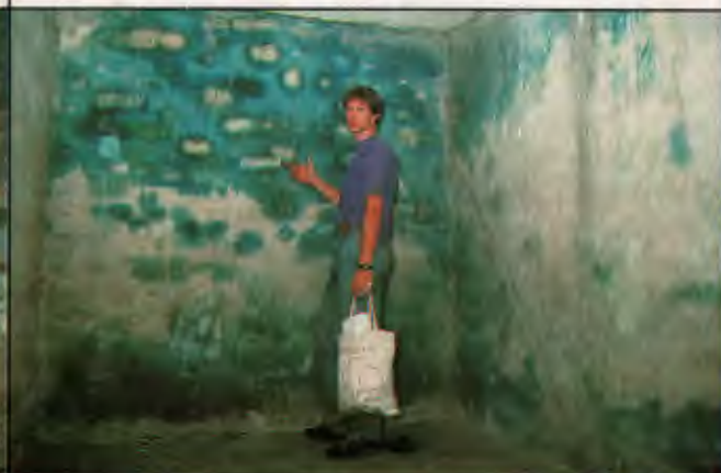
Illustration 9: Photo of the inside room located northwest of the delousing installation in building BW 5a. The outside wall with its intense blue pigment, caused by «Prussian blue», is visible in the background and right.
