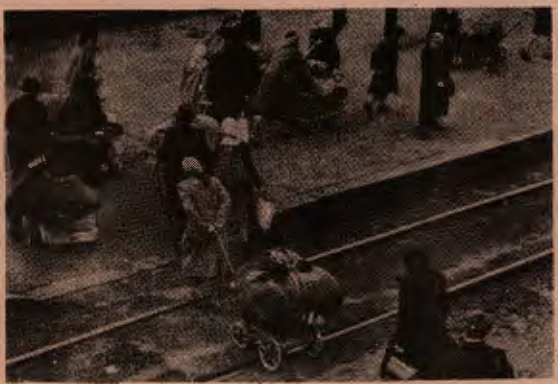
Refugees pouring into Dresden at the Central Station just before the raids!
