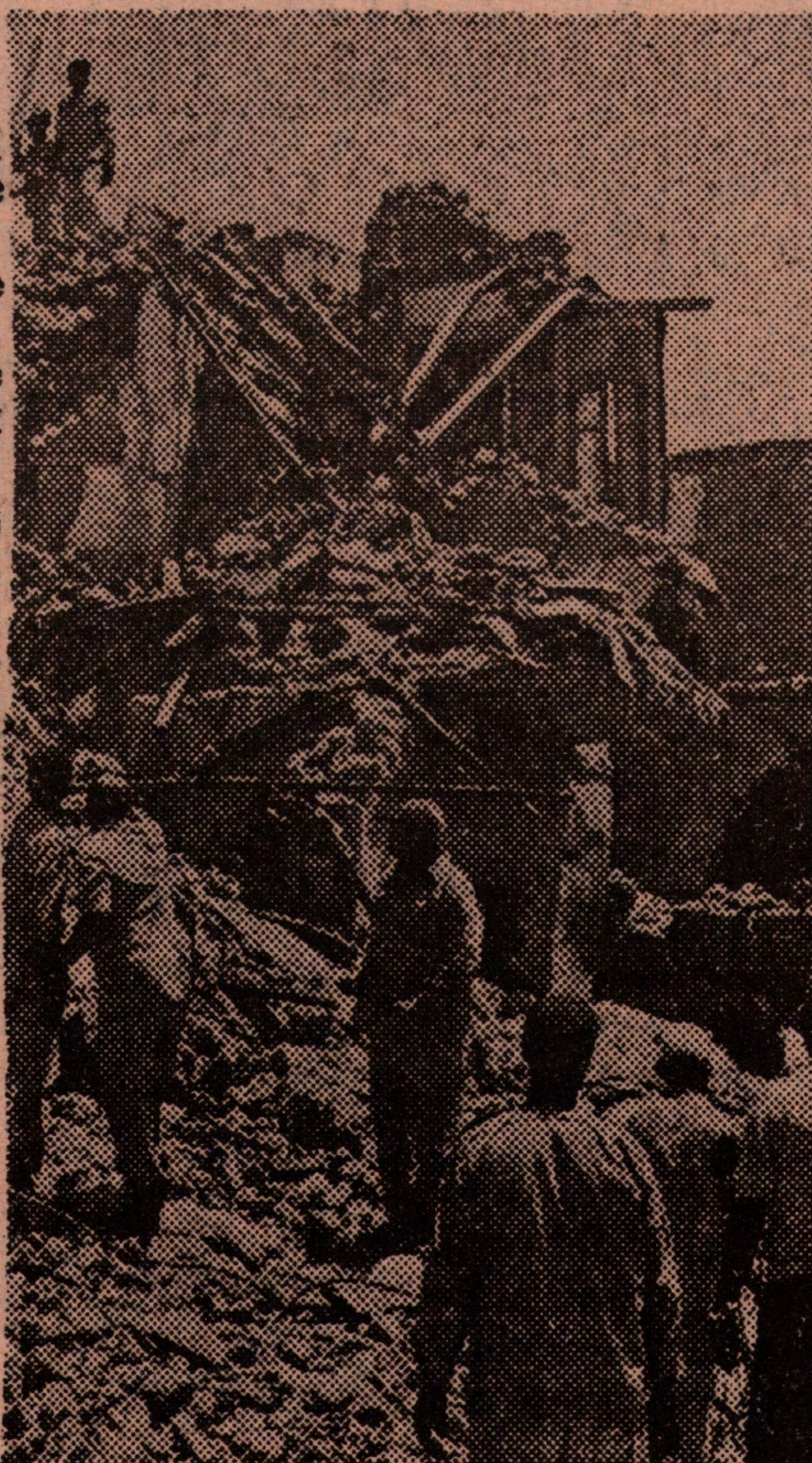
This apartment building in Cairo collapsed. 43 inhabitants died.
