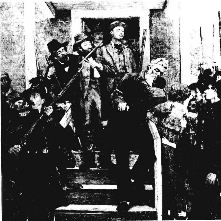
John Brown on his way to the scaffold
